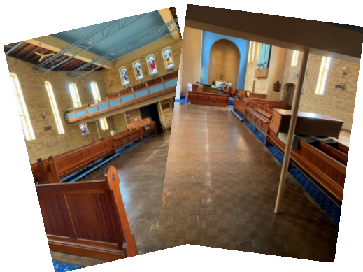
Church empty for repair work
