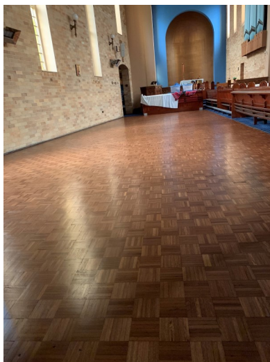
Parquetry flooring restored and polished
