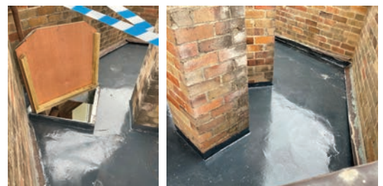
New manhole cover and waterproofing
