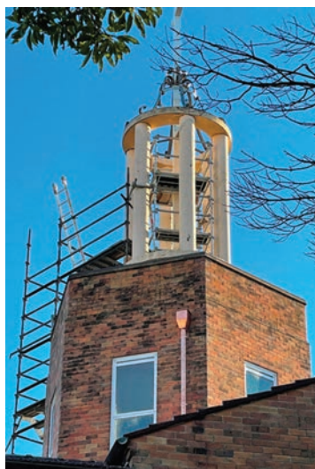
New copper rainwater head and downpipe
