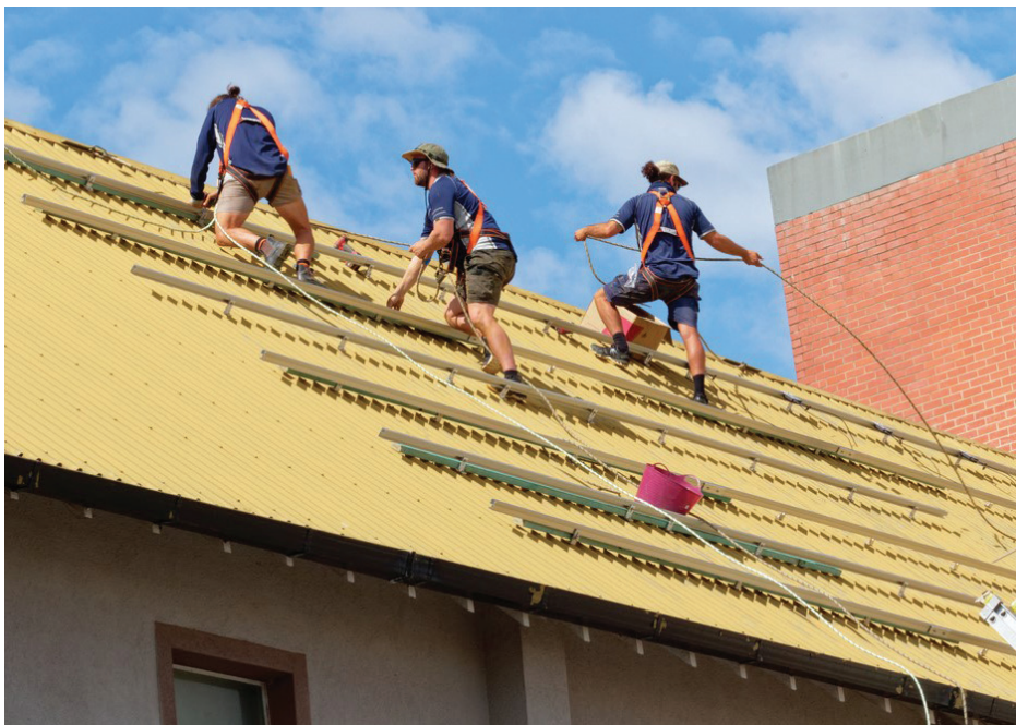
Installing brackets and climbing ropes
